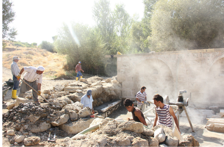
Construction at the Upper Fountain
